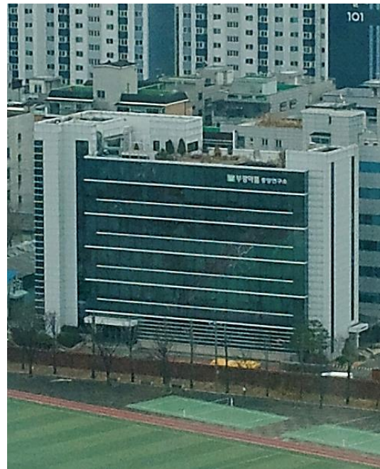
Facilities R&D Center Location 7, Sangdo-ro, Dongjak-gu, Seoul
